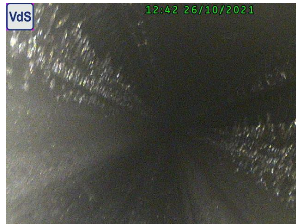
Typical air - water line
