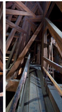
The attic, known affectionately as the "forest", it was made of 1.300 interlocked wooden beams, each crafted from an individual tree planted as early as the 8th or 9th century.
