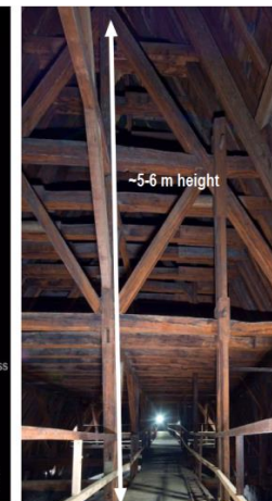
The attic, known affectionately as the "forest", it was made of 1.300 interlocked wooden beams, each crafted from an individual tree planted as early as the 8th or 9th century.
